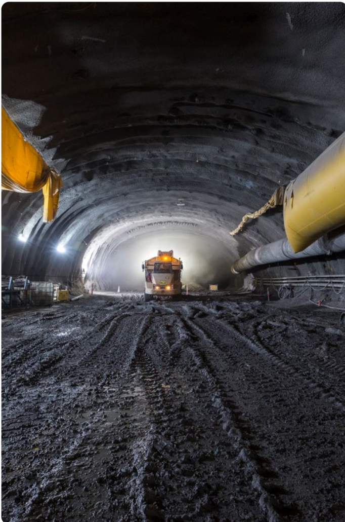
WestConnex - NSW, Australia
